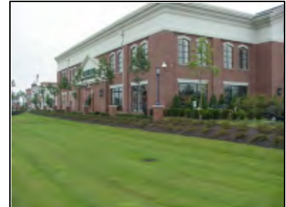
Brick building with appropriate window detailing.
