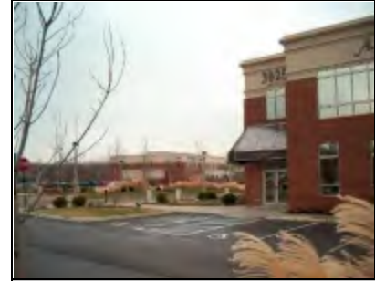
Two story office buildings with Awnings, Landscaping and Architectural detailing.
