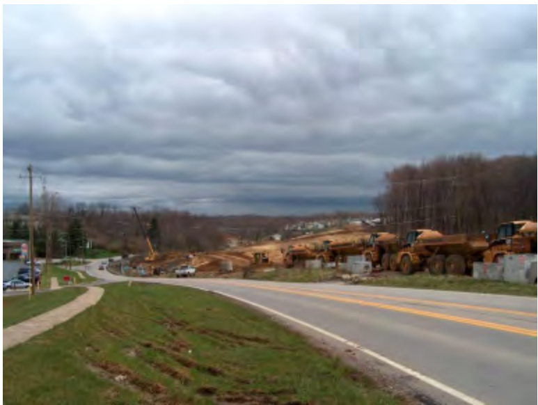
Road construction along Turkeyfoot Road near Florence, Kentucky. Source: Woolpert, Inc. 2006
