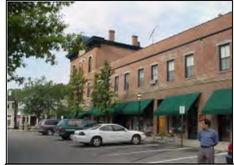
Consistent awning type and color unifies the façade.
