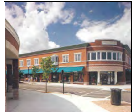
Commercial building with brick façade and appropriate awnings.
