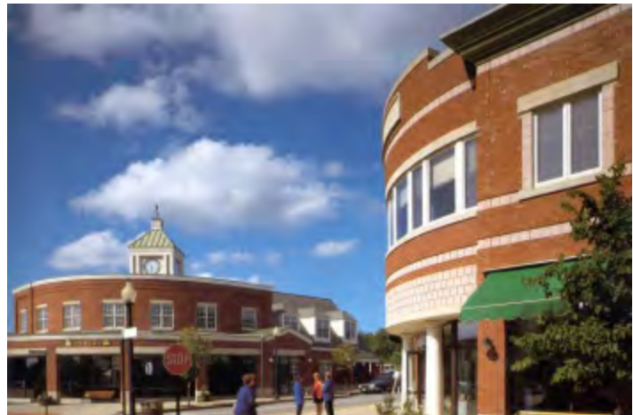
Suburban scale development- Mashpee Commons in Cape Cod, Massachusetts. Source: The New Urbanism page 175.
