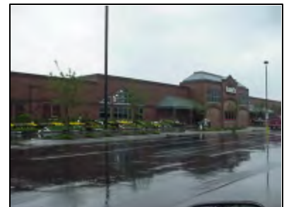
Large scale building example showing articulation of the façade.
