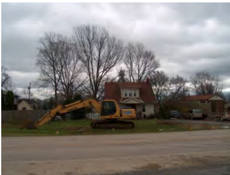
Road construction along Turkeyfoot Road near Florence, Kentucky. Source: Woolpert, Inc. 2006
