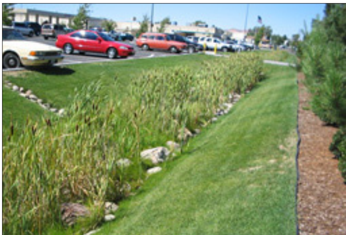
Figure 14: Retention pond and rain garden
