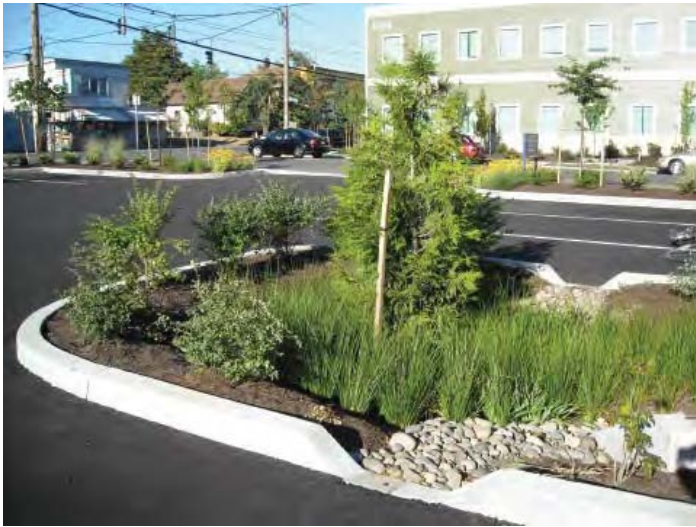
FIGURE 6.19 RAIN GARDEN/BIORETENTION AREA
