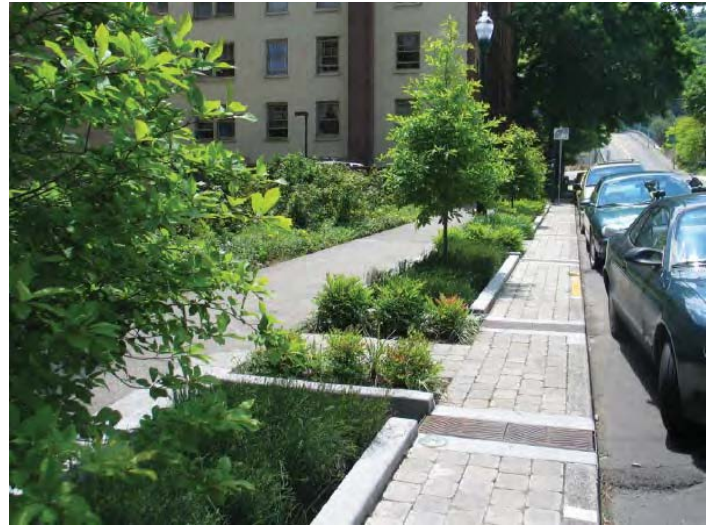
FIGURE 6.20 STORM WATER PLANTER BOXES
