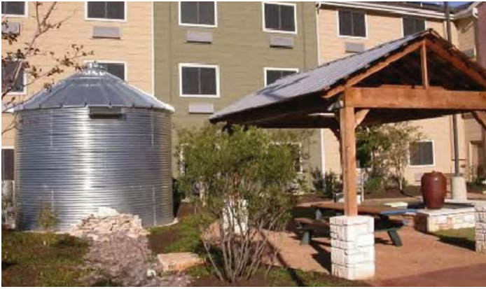
FIGURE 6.21 RAIN BARRELS AND CISTERNS
